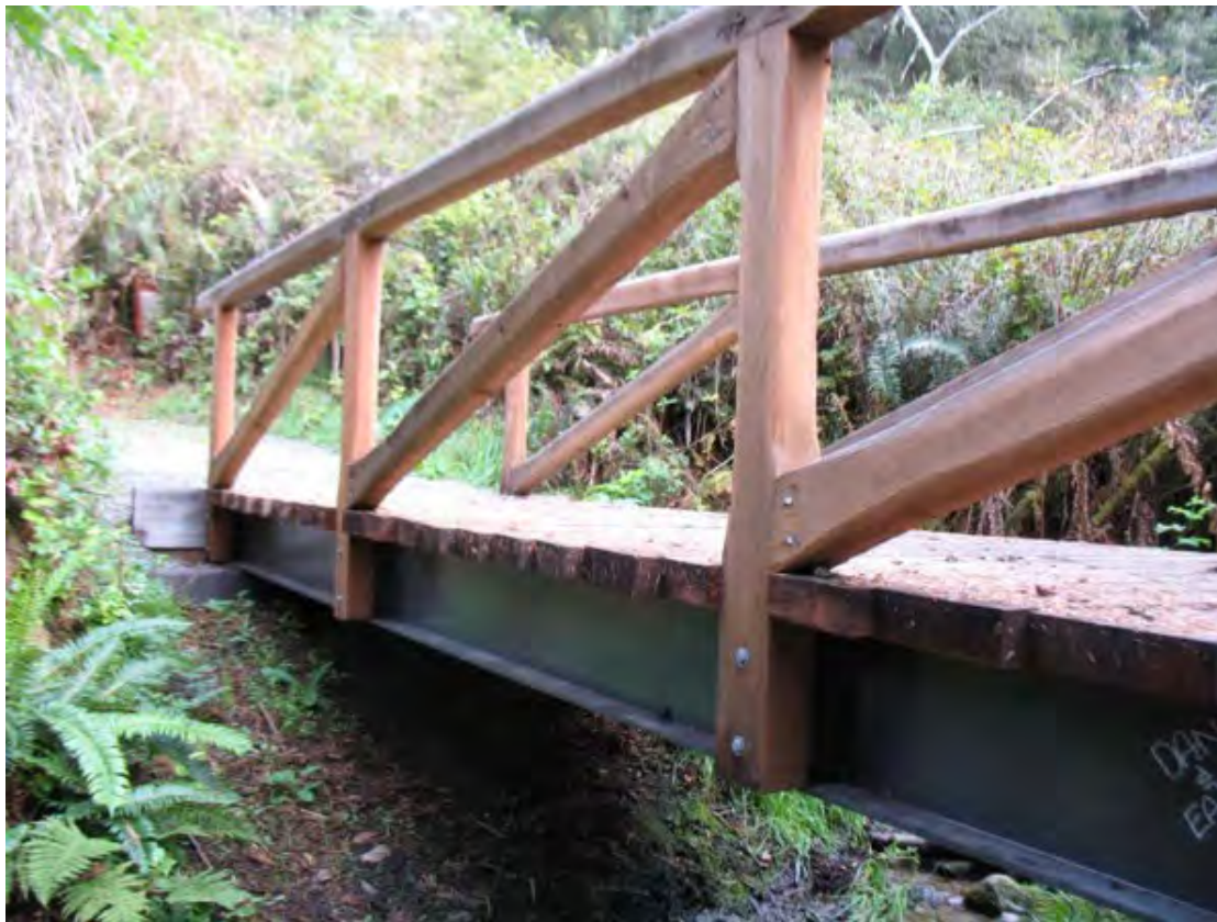
Typical Fiber-Reinforced Plastic Beam Bridge. Bridge shown here uses FRP stringers and redwood decking and railing. The bridges for the Montgomery Grove Project will be constructed entirely of fire-resistant FRP materials.
